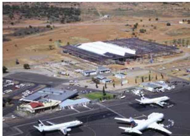
New terminal under construction
